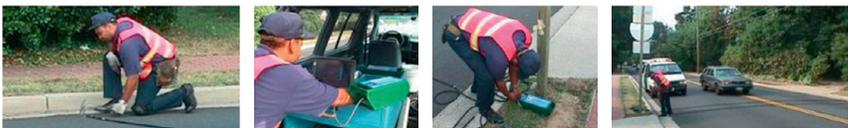
**Figure 1.4** Installation of pneumatic tubes. (Photos from <http://www.arlingtonva.us>.)
